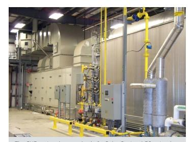
The CHP system is comprised of a Solar Centaur® 50 natural gas combustion turbine and a Rentech HRSG equipped with supplemental duct firing. Photo credit Frito-Lay North America, Inc.
