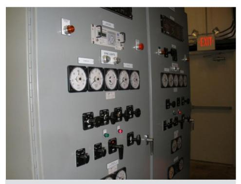
The Frito-Lay plant has electrical interconnect, including switchgear, primary power wiring, relays, etc., allowing power generation in parallel with Connecticut Light and Power's electrical grid. *Photo credit Frito-Lay North America, Inc.*
